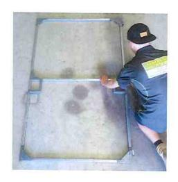
2. Measure your opening and if required, make simple, straight cuts to alter gate height/width.
