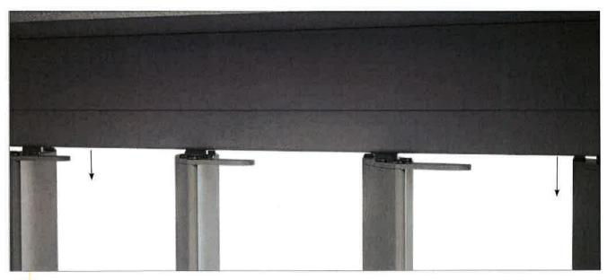
Once all Louvre Blades are inserted, remove clamps and carefully lower the Top Rail so that it sits on the top pins.
